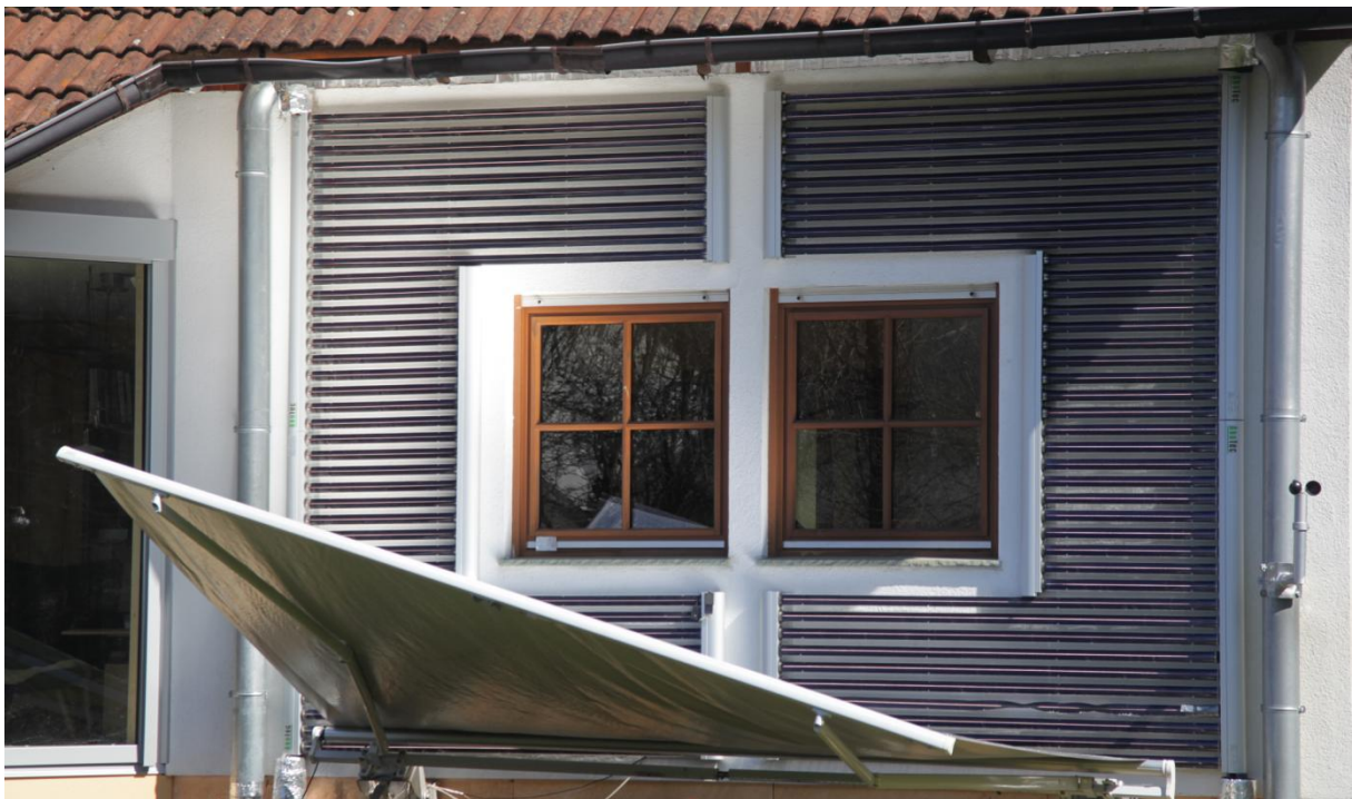
Figure 6: Stahrsolar - collector with positioned reflector
